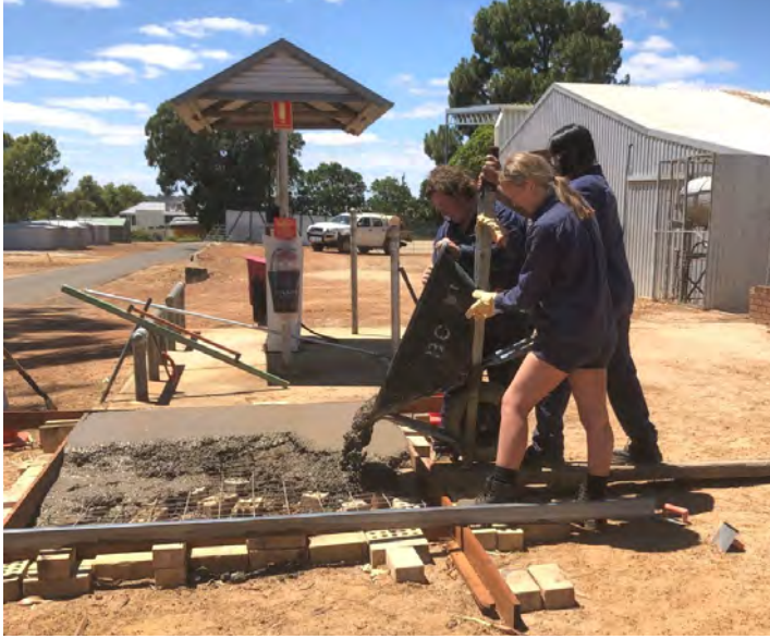
Year 12 Students laying a concrete slab for the new fuel bowser.
