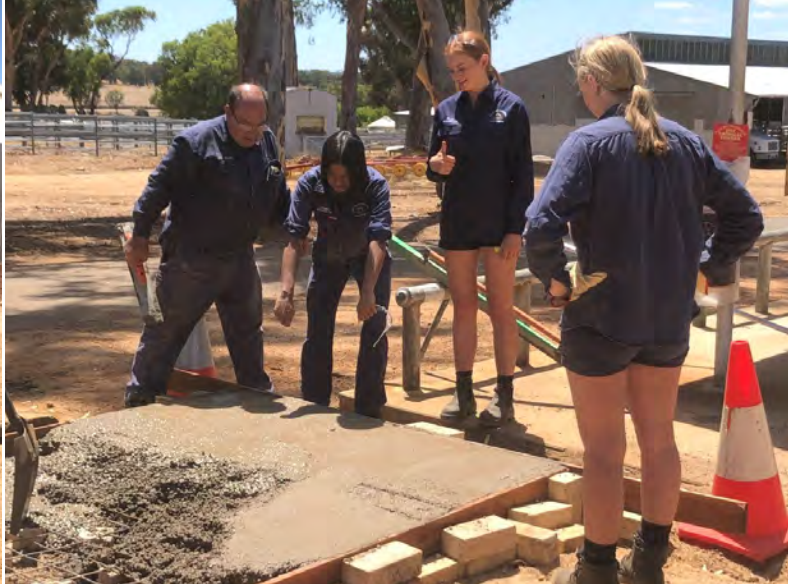
Year 12 Students laying a concrete slab for the new fuel bowser.
